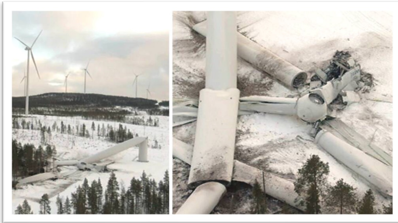
Aldermyrberget, Sweden, November 2020
