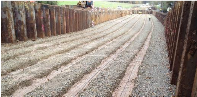
Installation of sensing cables
