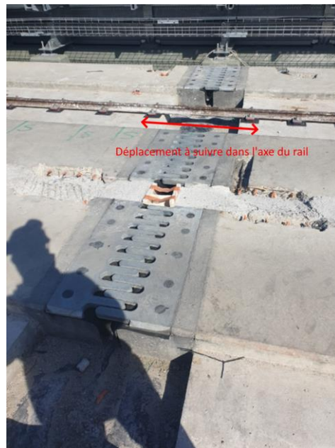
Joints de dilatation
