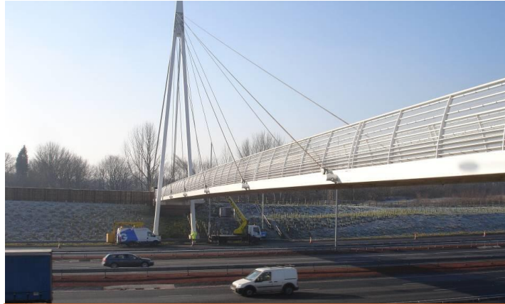
INFRASTRUCTURES GENIE CIVIL
